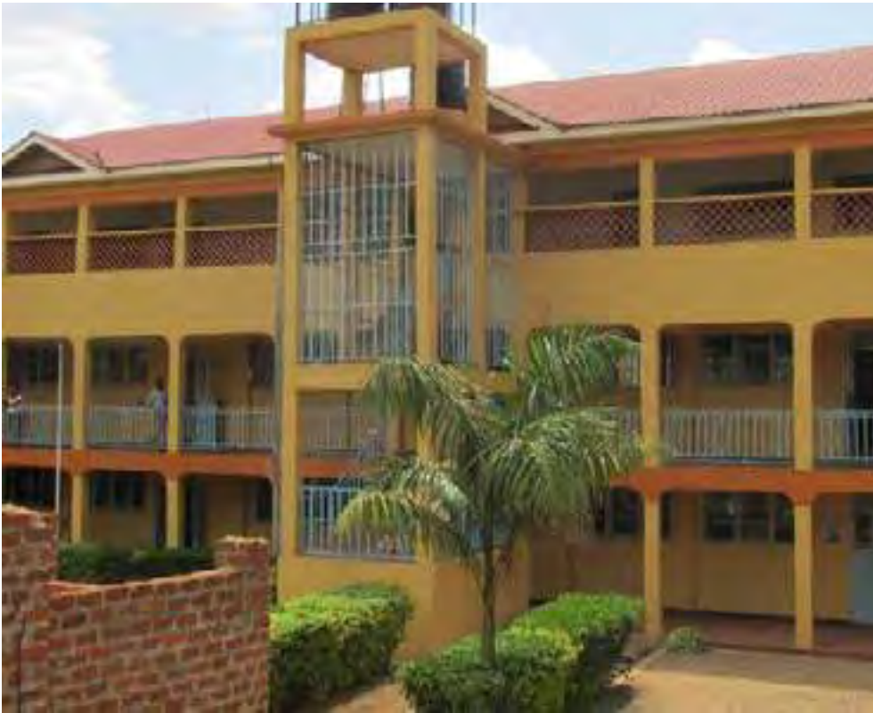
Above is the Faculty block at Mbale
