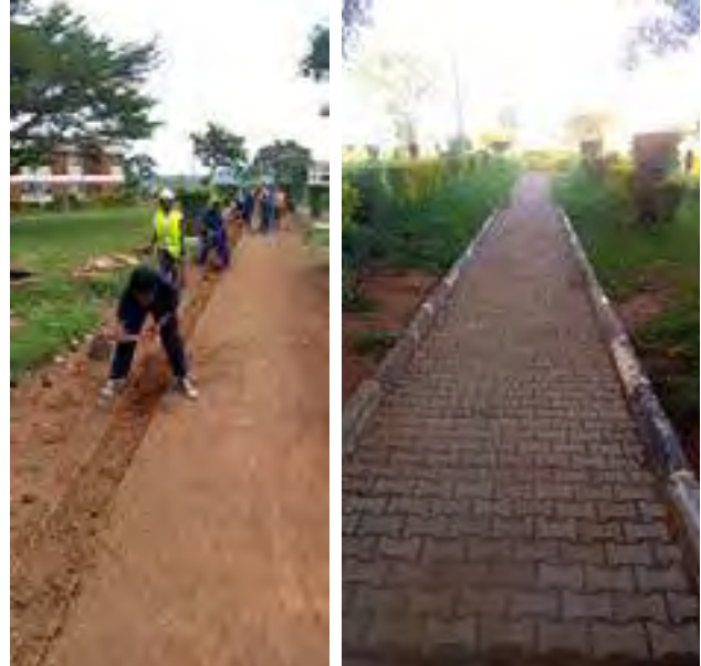
Walkway to Main Administration Block
