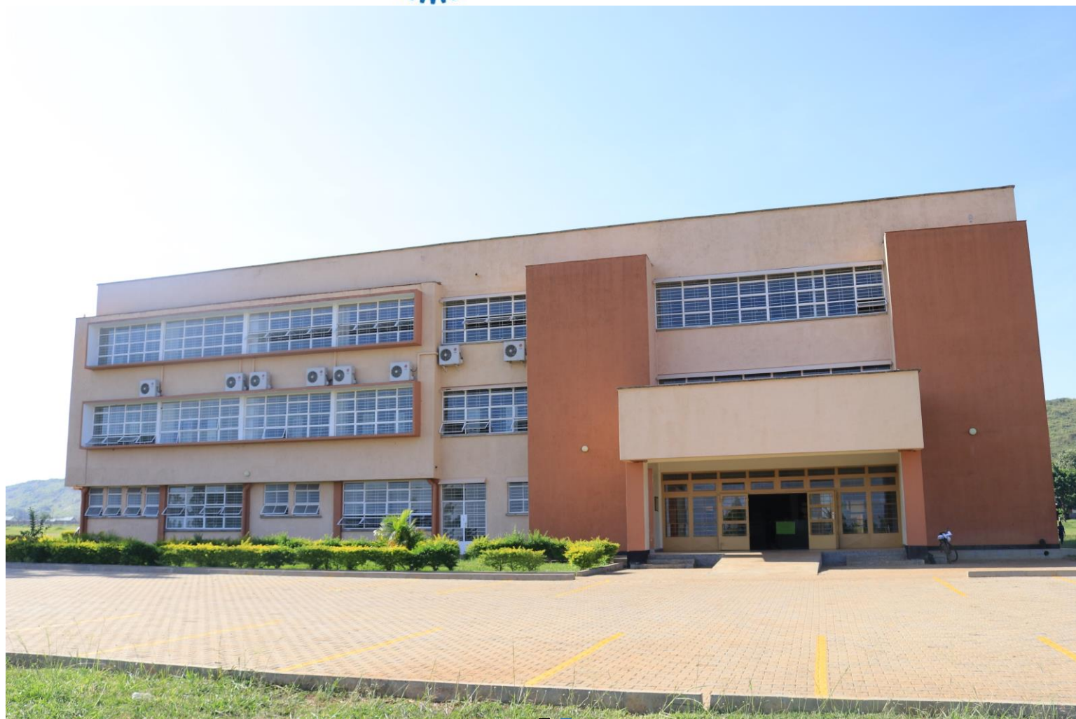
Engineering Library @ Busitema – Front View
